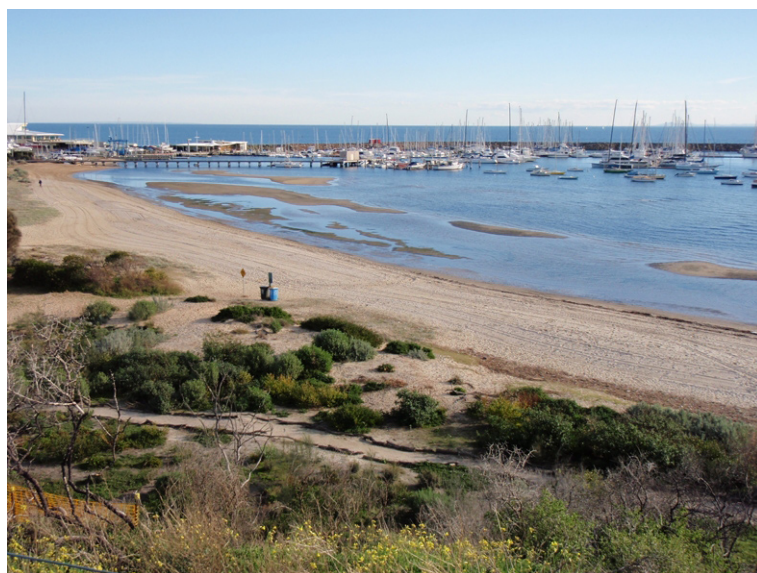
At Sandringham harbour the prevailing winds move sandy sediments along the coastline either northwest or southeast depending upon the season. Changes to coastal engineering have affected this geomorphic process. Sand is trapped behind the groyne causing the harbour to shallow over time.
